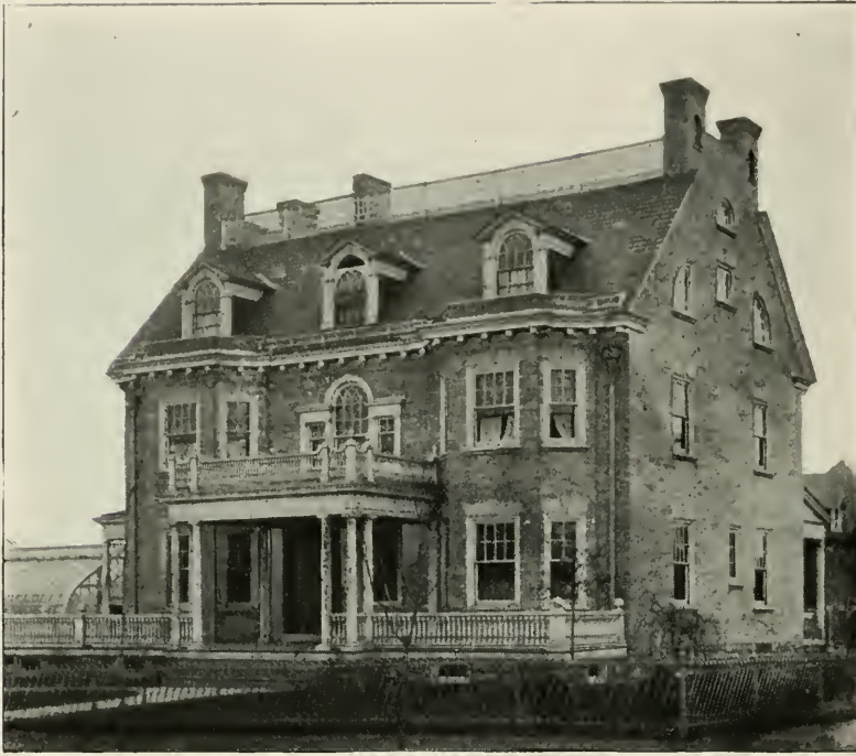
RESIDENCE OF D. G. DERY.
