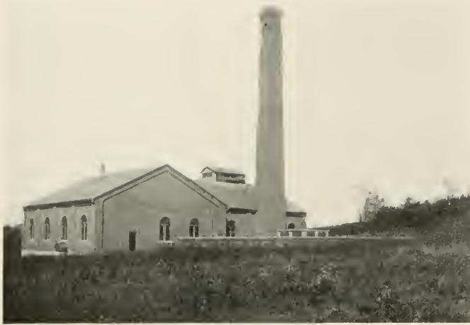
THE PUMPING STATION.
