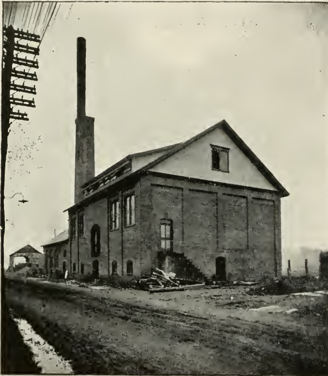
LEHIGH-NORTHAMPTON POWER HOUSE.
