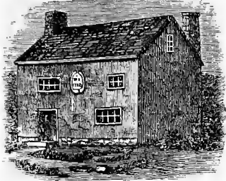
OLD SWEDE BUILDING
