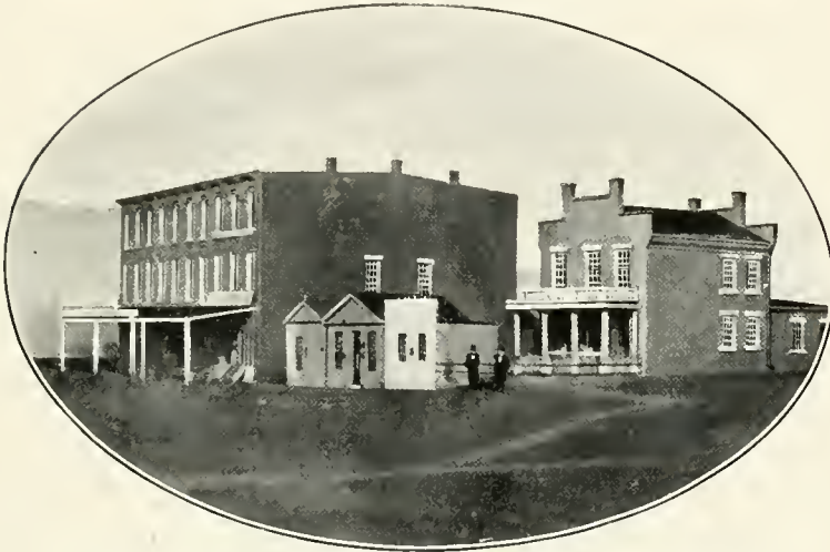
FRANKLIN BLOCK AND RESIDENCE OF P. W. EARLE First Brick House in Cedar Rapids
