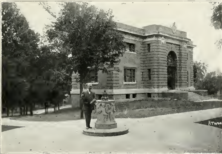
CARNEGIE LIBRARY AND SPEER MEMORIAL FOUNTAIN, MT. VERNON
