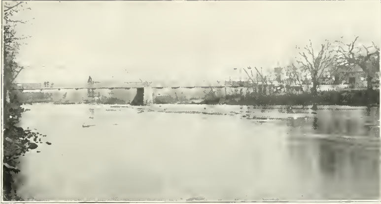
UPPER WAGON BRIDGE, CENTRAL CITY
