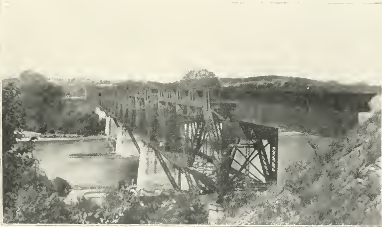
MILWAUKEE BRIDGE, AT COVINGTON
