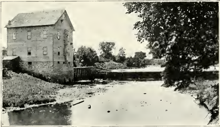
MILL AND DAM, COGgon
