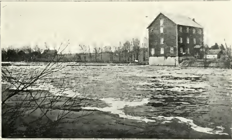
WAPSIE RIVER AND MILL Built in the '50s at Central City
