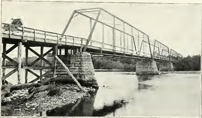
BRIDGE OVER CEDAR RIVER AT CENTER POINT
