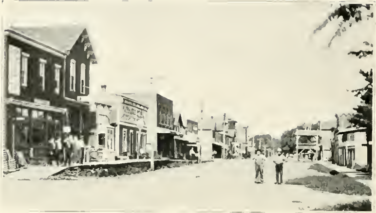
MAIN STREET, CENTRAL CITY, FROM THE SOUTH
