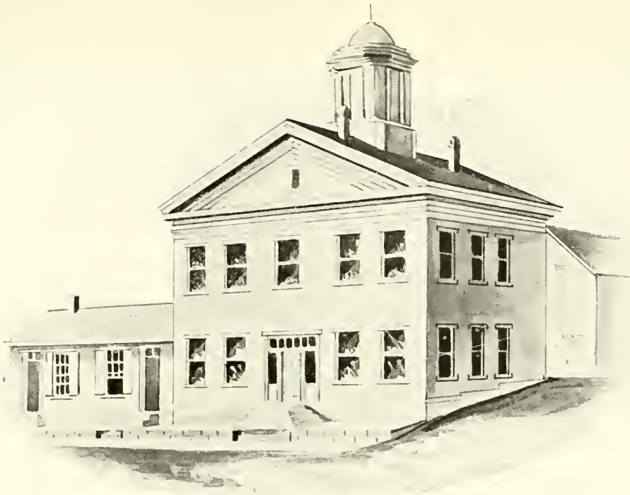
PIIONEER COURTHOUSE AND JAIL, 1831
