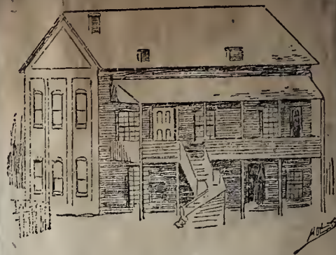
Old Schoolhouse, Robinson Street.
