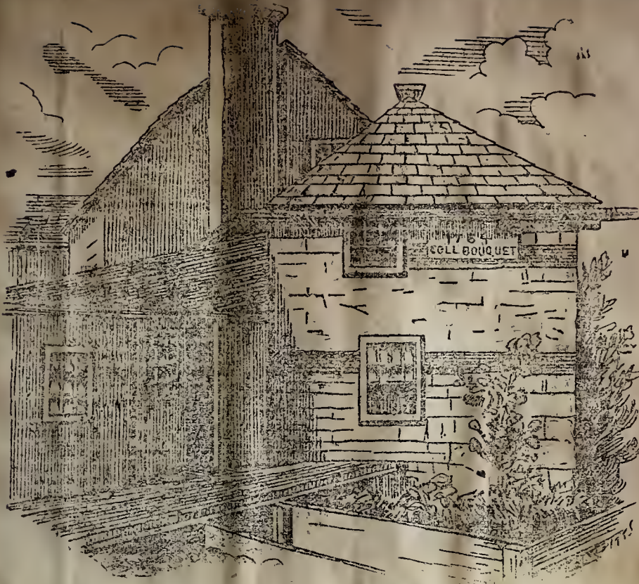
THE OLD BLOCK HOUSE.
