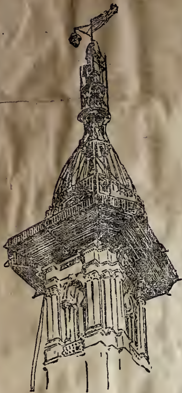
HOISTING THE HEAD AND HAT INTO POSITION.
