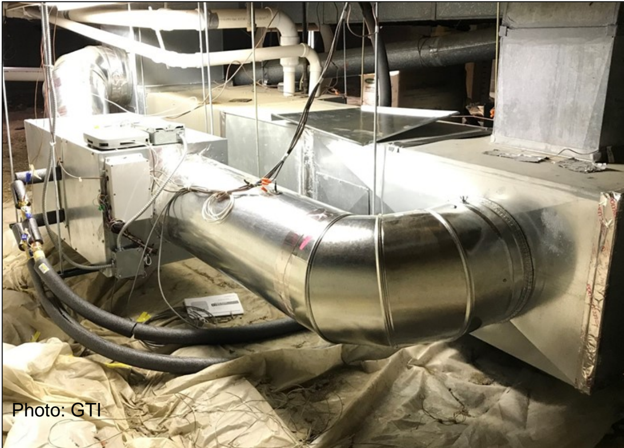
Horizontal install (parallel to existing furnace for pilot)
