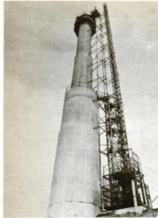
The tower of the **Tvind** windmill is over 50 metres high—the rotor axle is 54 m above ground level. When finished the windmill will generate up to 2 megawatts of electrical output and 3600 MWh/yr. There will be two 27 m long blades. The maximum usable wind speed will be 14 m/s, and the maximum rotor speed 40 revs/min when the blade tips will be travelling at 400 km/h
