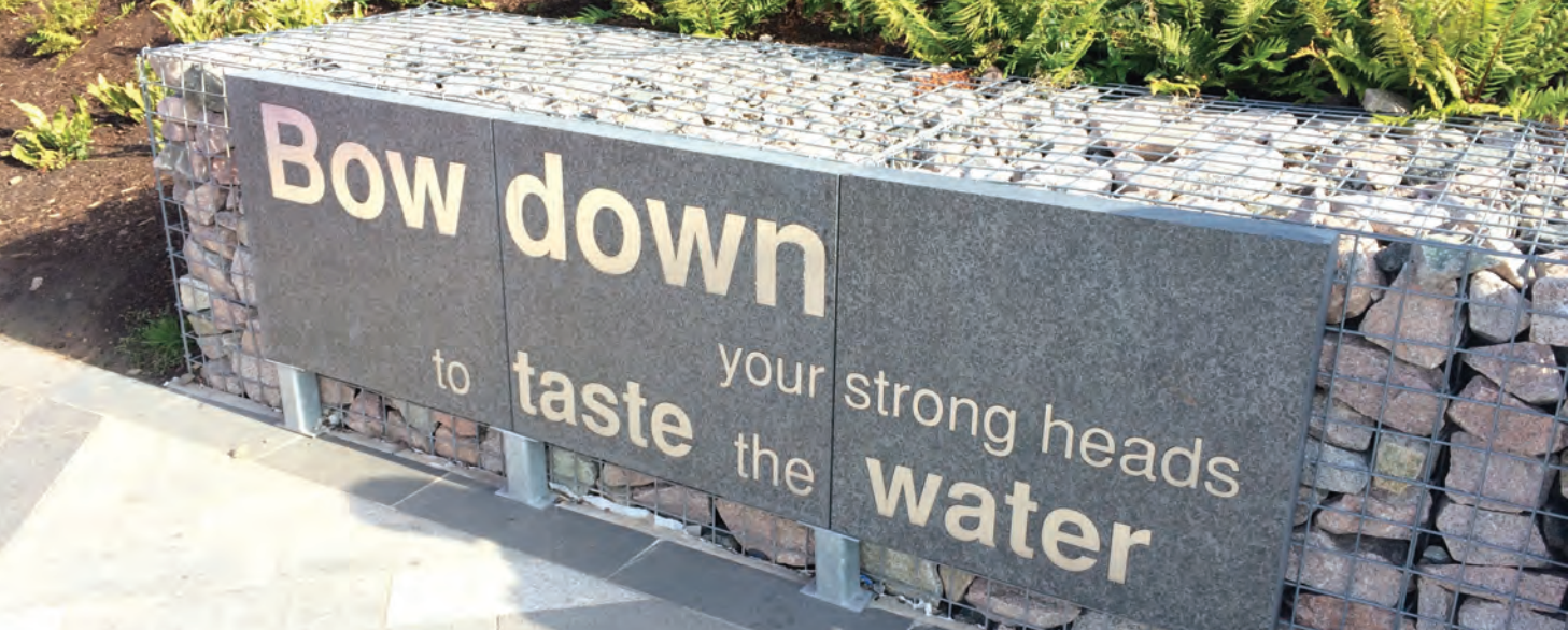
Example of signage fixed to gabions
