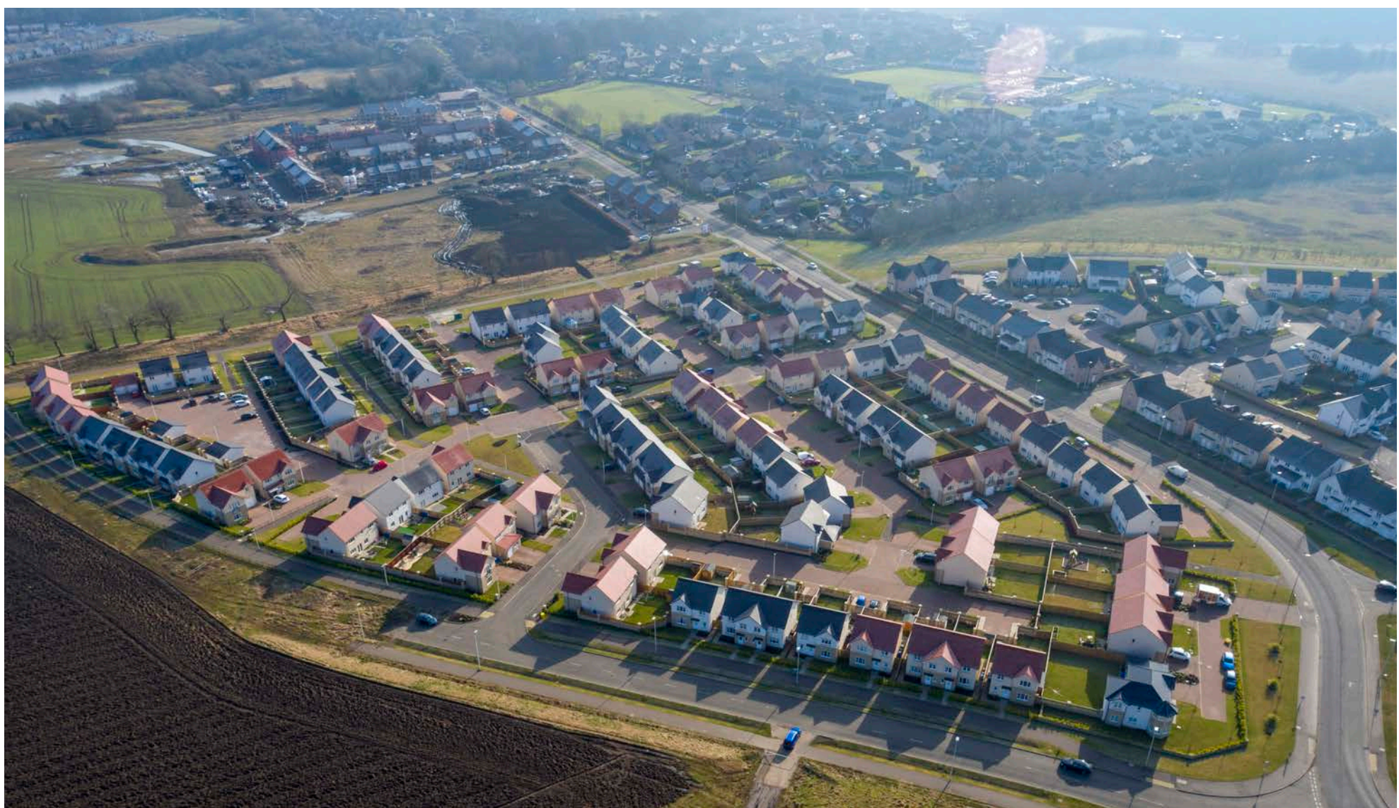
Aerial view of new housing in Winchburgh.
