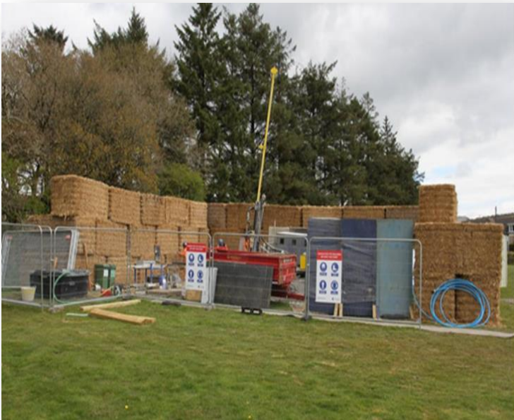
Diamond drilling in progress
