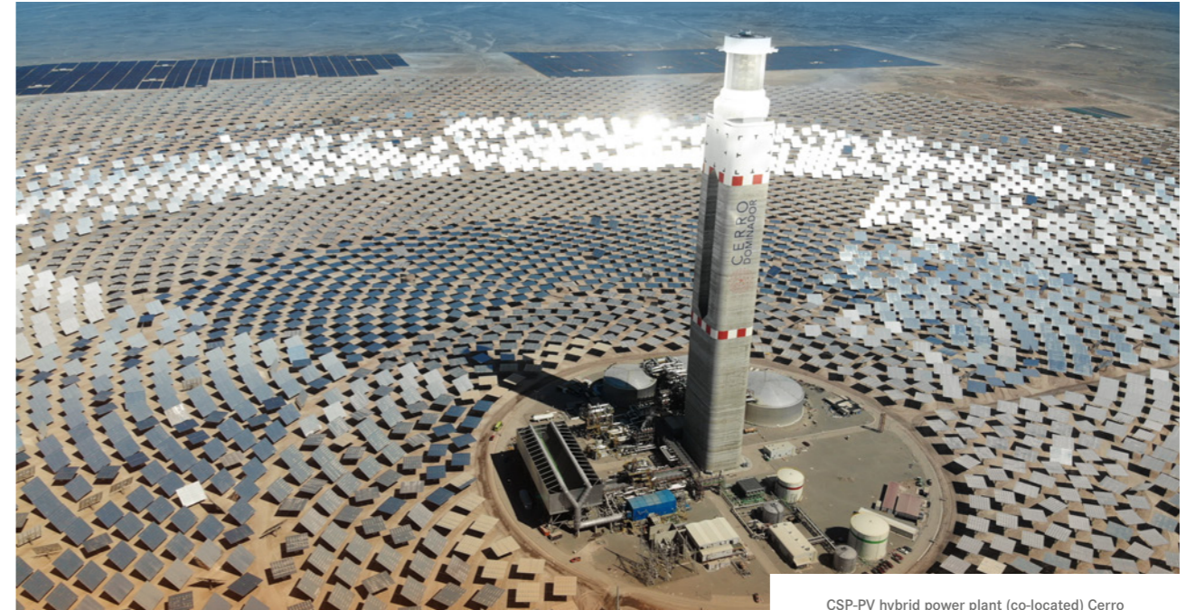
CSP-PV hybrid power plant (co-located) Cerro Dominador, María Elena/Chile (CERRO DOMINADOR)
