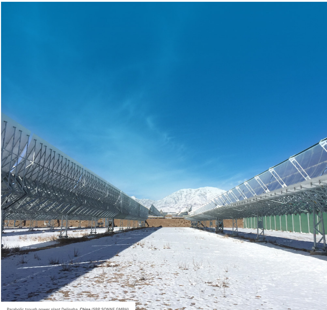
Parabolic trough power plant Delingha, China (SBP SONNE GMBH)
