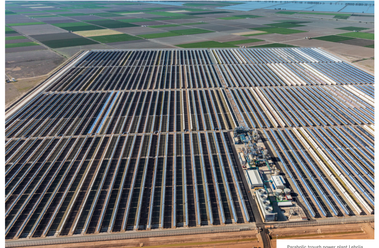
Parabolic trough power plant Lebrija, Spain (SIEMENS, 2012)
