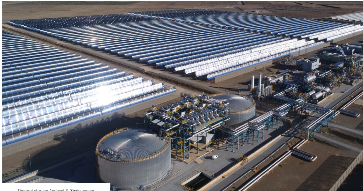
Theramli storage Andasol 3, Spain, owner Marquesado Solar (CSP SERVICES GMBH)
