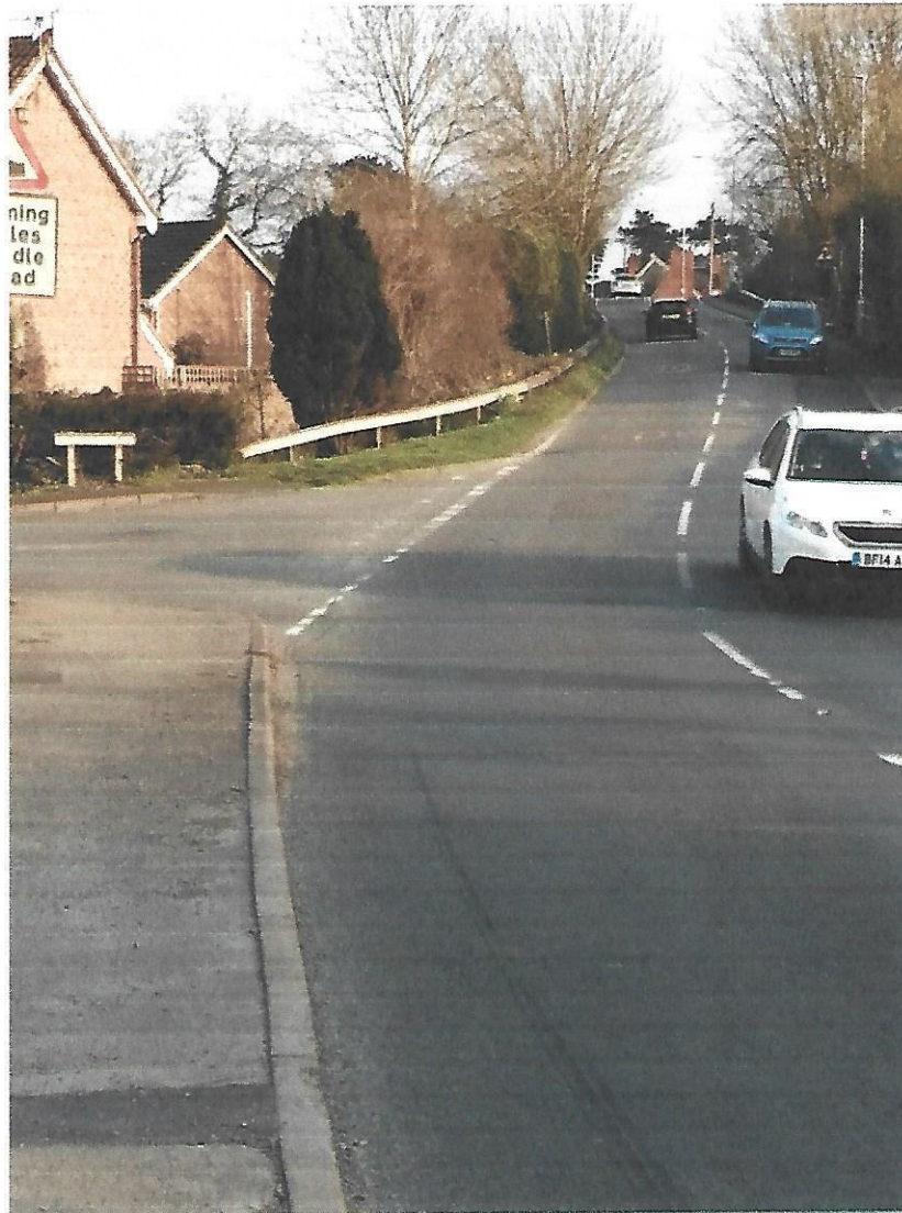
Photograph 4 – B581 Station/Stanton Road Railway Bridge at Bostock Close junction
