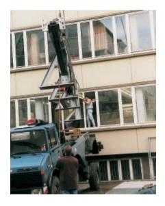
The machine was dimensioned so that the width and the length corresponded to the available space through the window as well as floor length in the factory.
