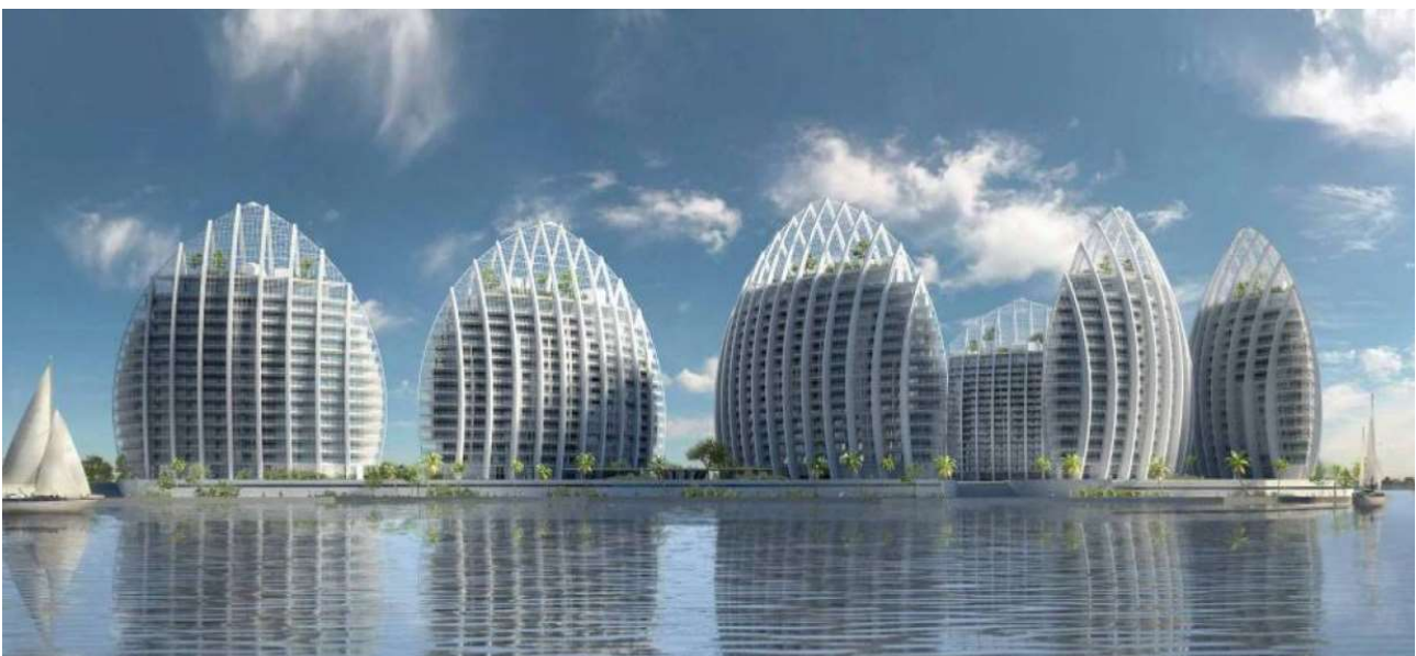
Putrajaya Waterfront Residential Complex – Kuala Lumpur, Malaysia Source: Studio Nicoletti Associati
