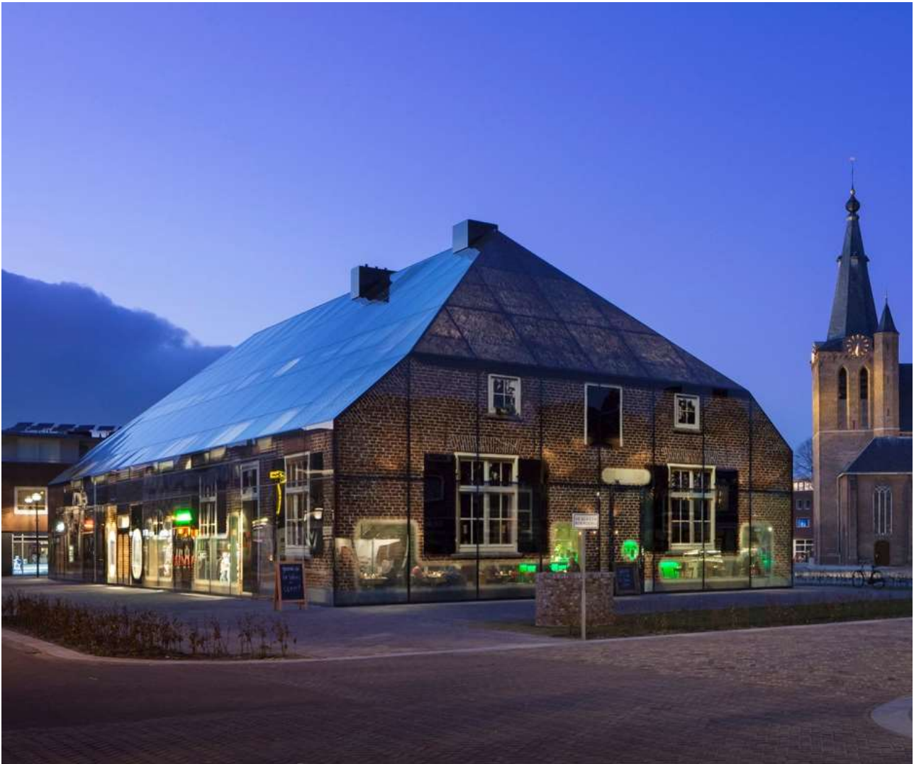
Glass Farm Schijndel Source: MVRDV
