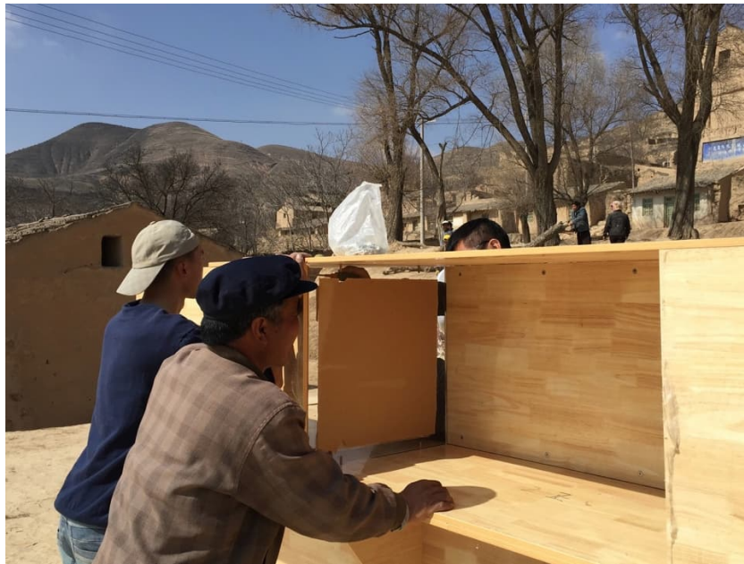
Figure 5. Worker positioning a plywood panel shortly before the cam-locks are fastened
