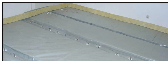
installed shear connectors and timber beam ceiling covered with PE-foil
