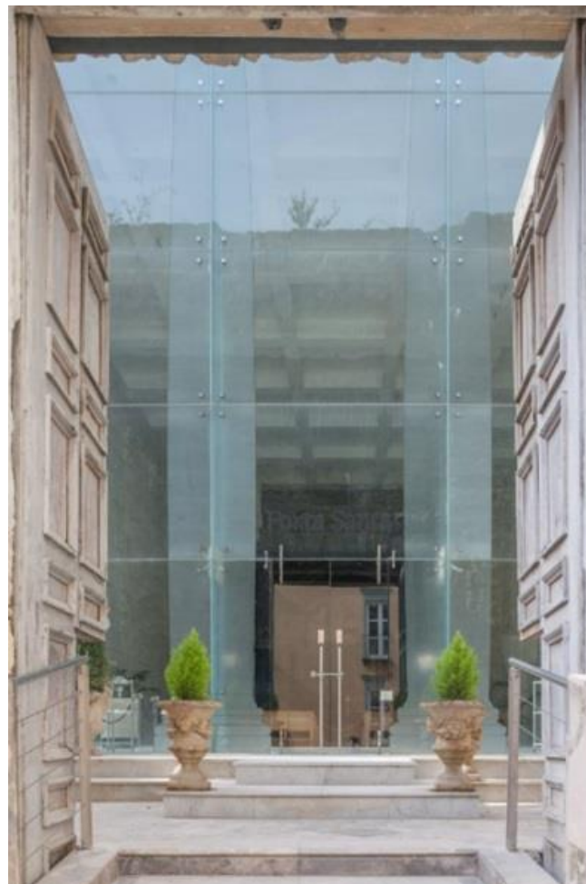
Figure 2. The new glass facade, showing the glass columns
