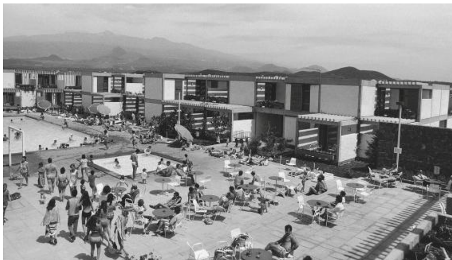
Figure 6. Díaz-Llanos/Saavedra & Cabrera: The Drago apartment ensemble. Photograph: ©E. Pintos
