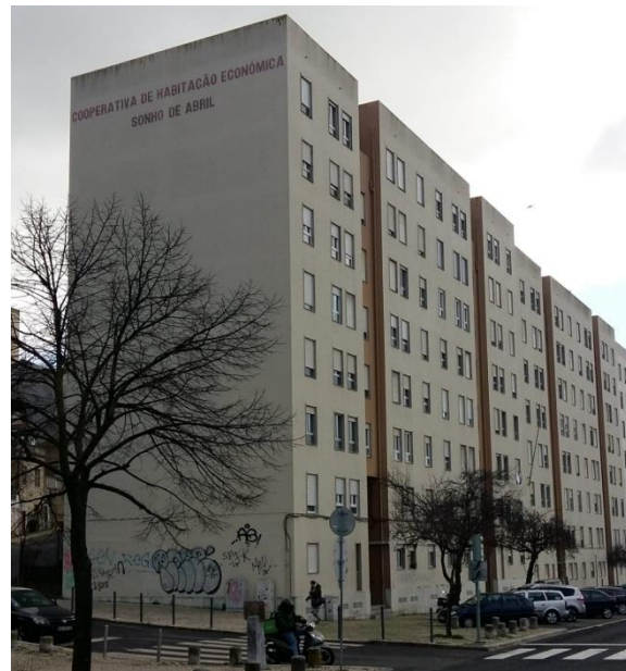
Figure 12. Housing blocks for the rehousing of shanty town's inhabitants, 1980's
