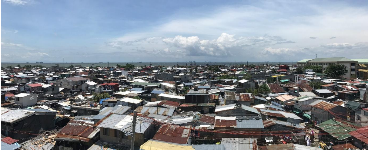
Figure 7. BaSECo District in the Port Area of Manila.
