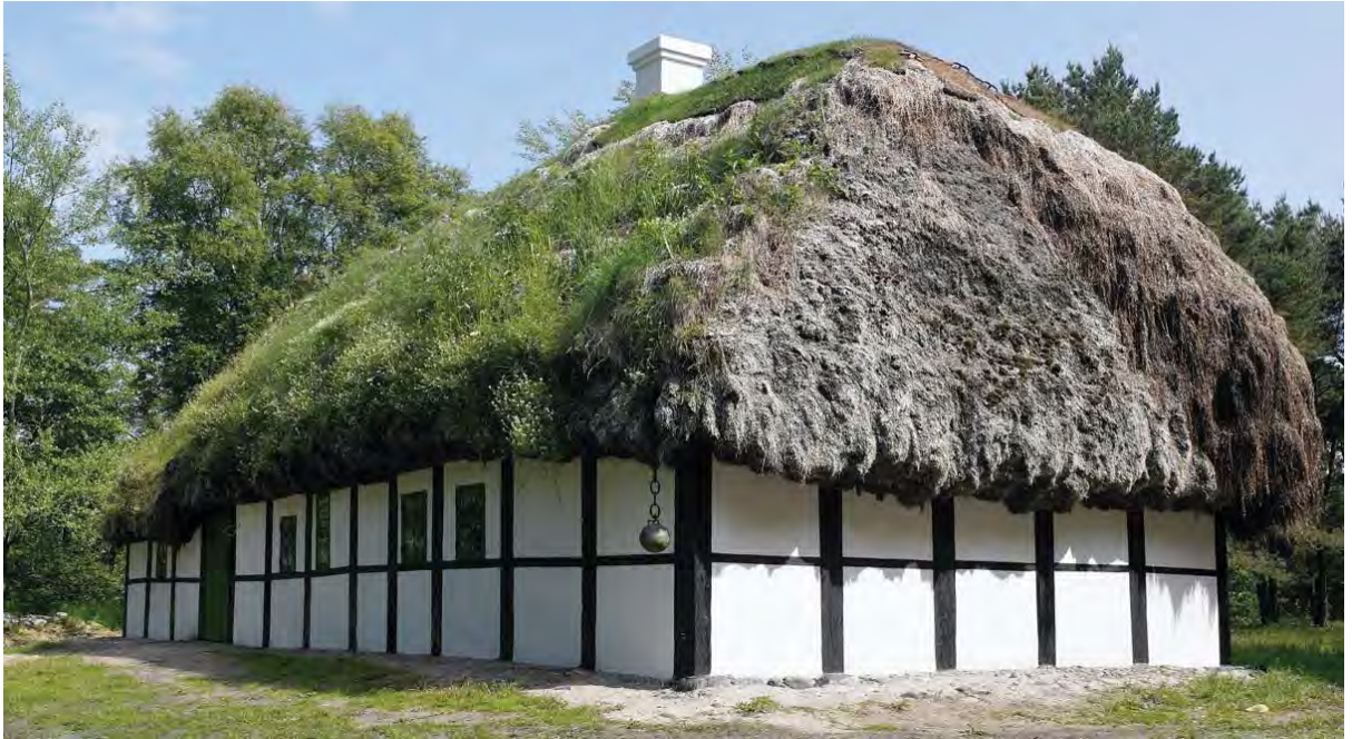
Figure 2. Photo of eelgrass roof, Kaline's House, Læsø. Photocredit: Helene Høyer Mikkelsen.
