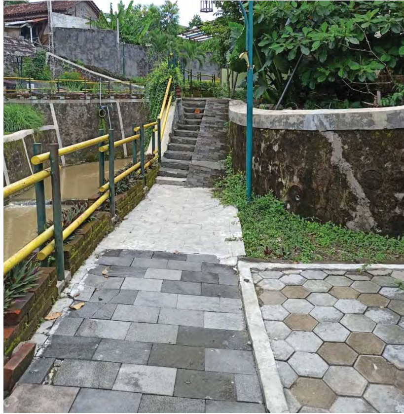
(Figure: Karangwaru riverside street condition with paving block pavement)
