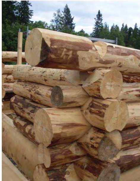
Figure 4. Corner of Laft timber construction. Photocredit: Norges Husflidslag.
