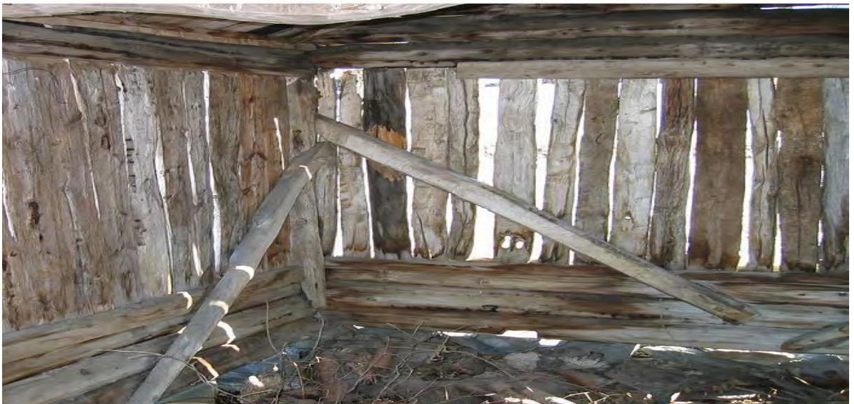
Figure 5. Timber wall of vertical planks ( stav ). Photocredit: Northhouse.org.
