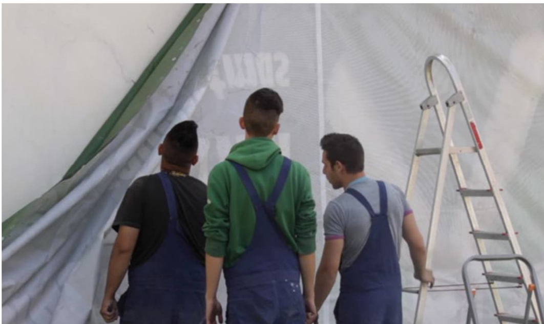
Figure 6. Installation of construction safety net
