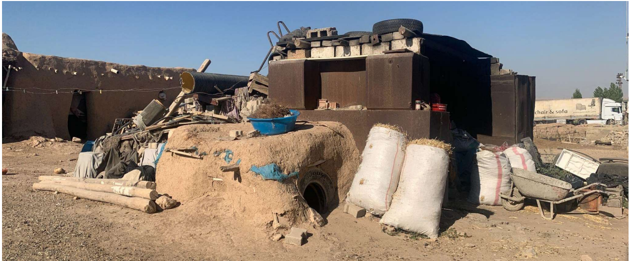
Figure 12. Tandoori and poultry complex from fuel tanks, tires and mud (also Figure 1)
