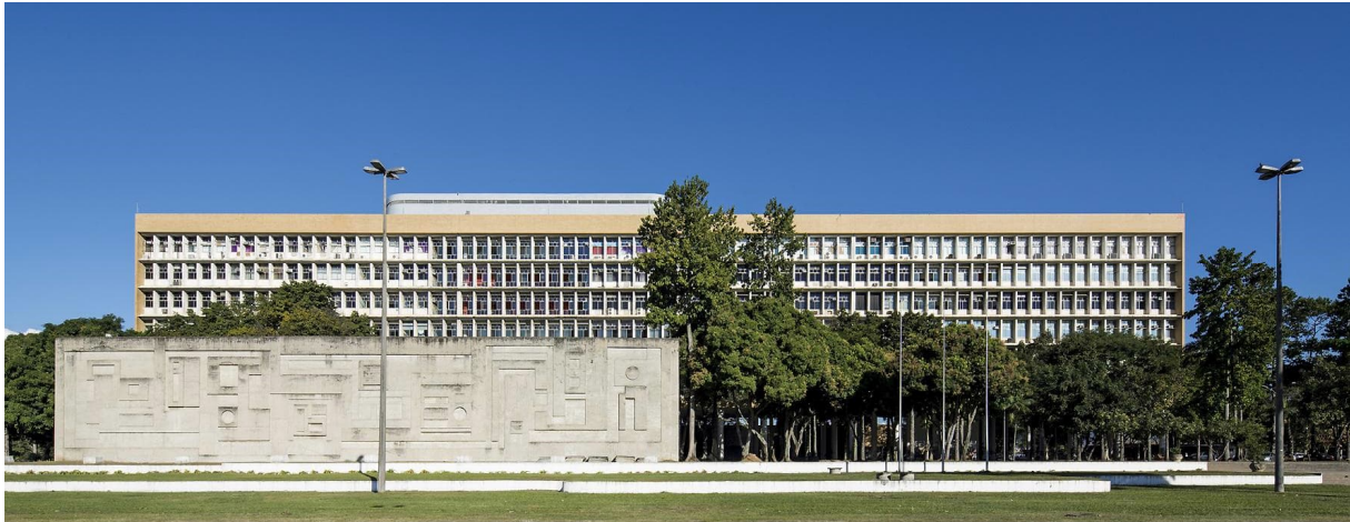
Figure 6. JMM Building façade with Burle Marx panel in 2015 Photo by Andréa Borde.
