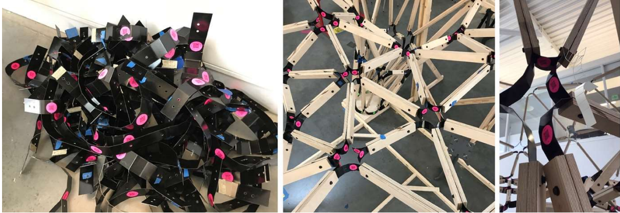
Figure 05. QR codes applied to unique parts for identification and easy of assembly.
