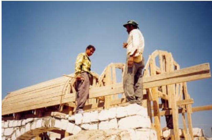
Figure 4. Wooden formwork used in construction
