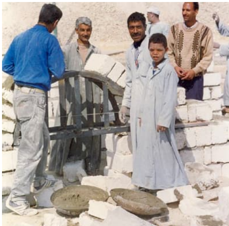
Figure 5. Training of workers on the construction method
