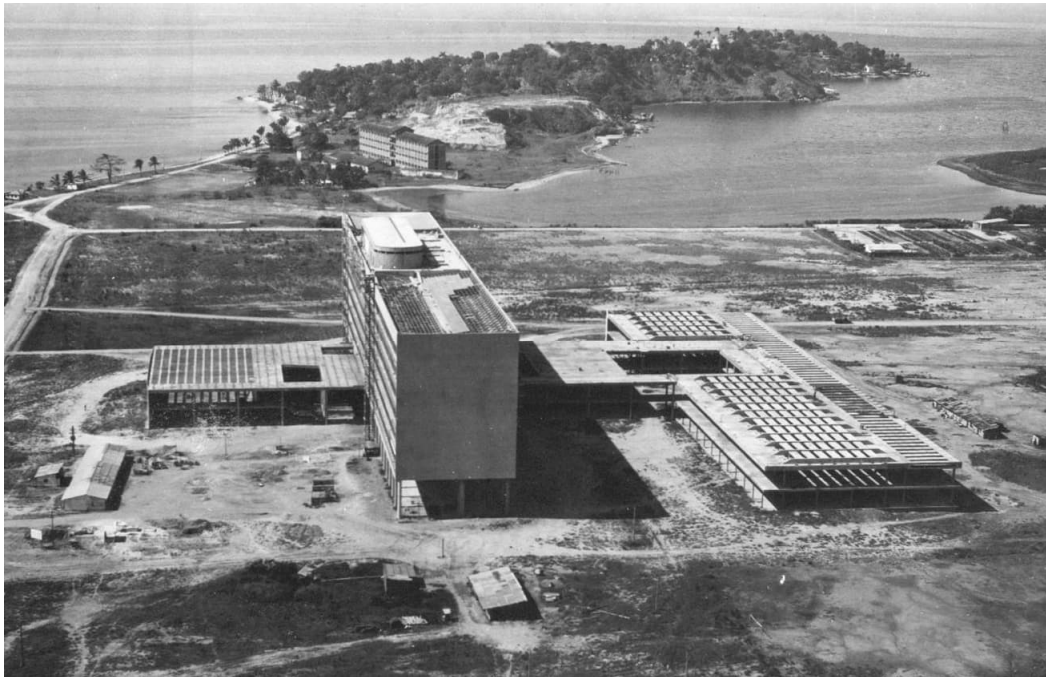
Figure 2. The JMM building, former headquarters of the FNA, under construction in 1959.
