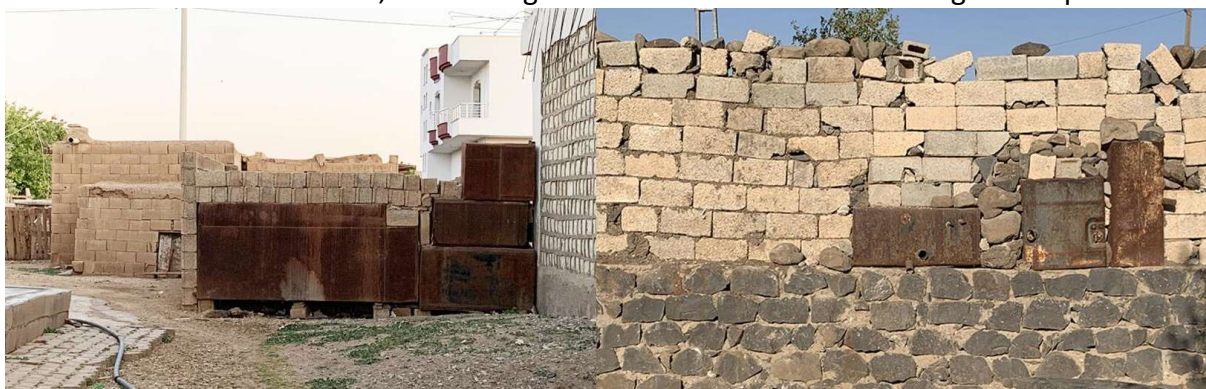
Figure 7. Fuel tanks used as bricks. Left: Boztepe, Right: Okcu
