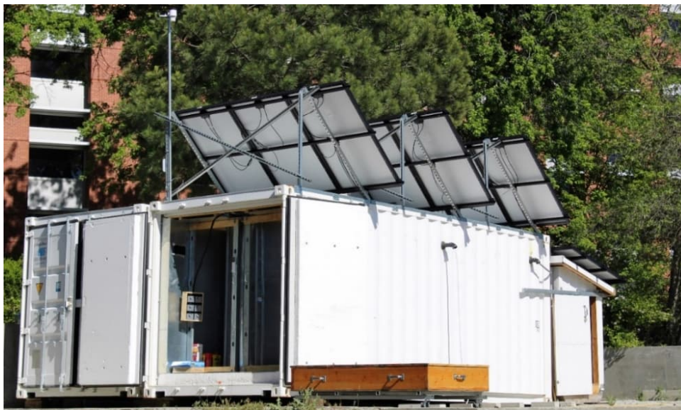
Figure 1: Test chamber overall construction photo from the northeast corner of the site.
