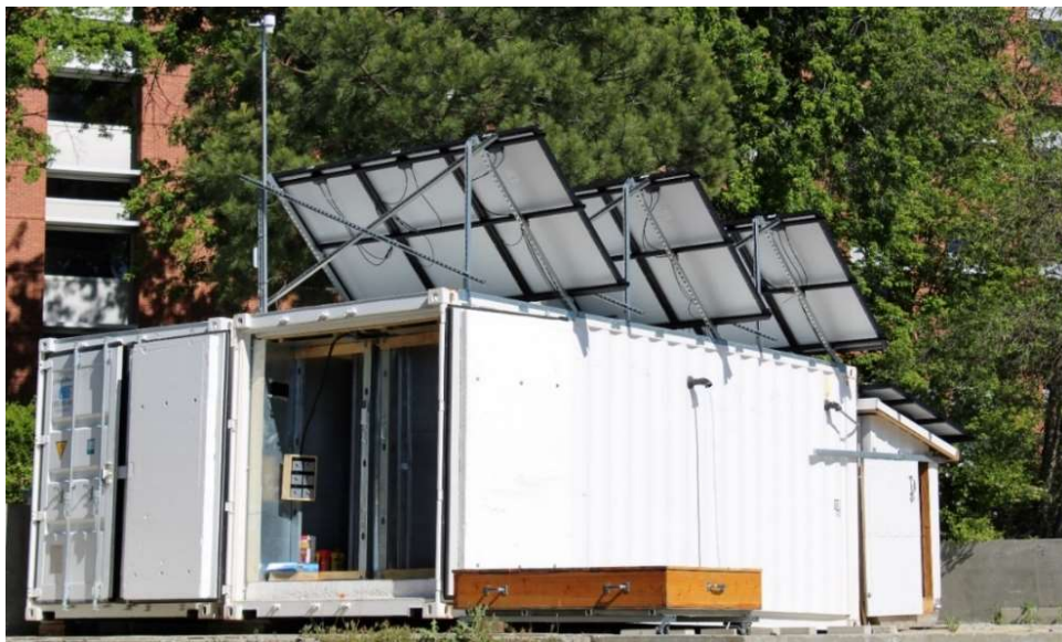
Figure 1: Test chamber overall construction photo from the northeast corner of the site.
