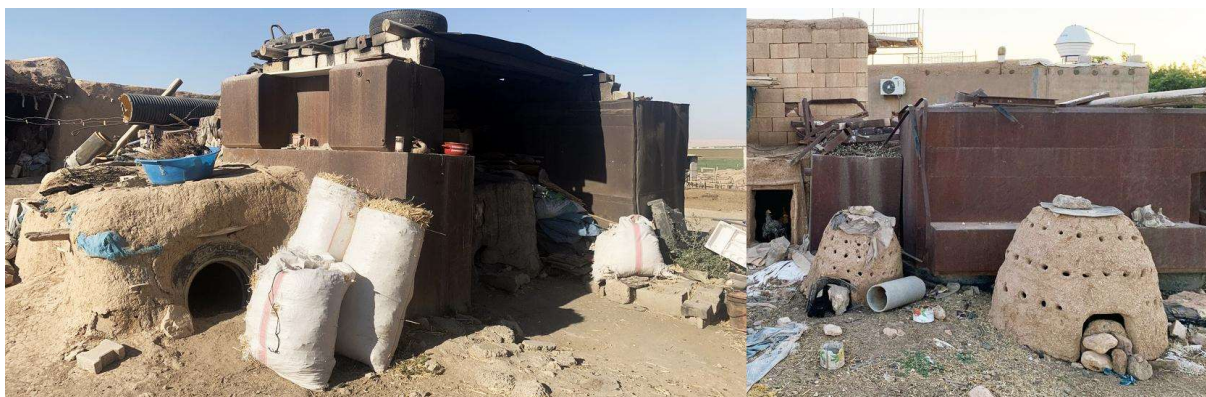
Figure 8. Fuel tanks integrated with mud. Left: Calıslı, Right: Boztepe
