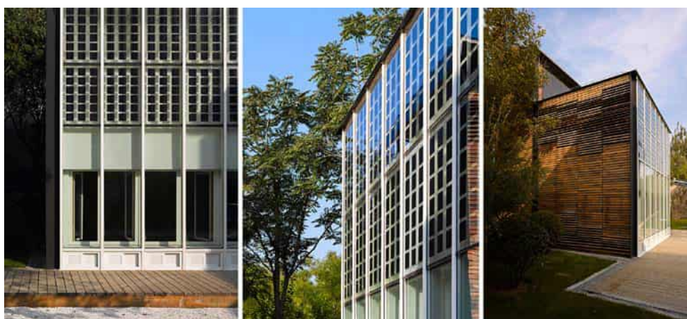
Figure 5. Application of DSF prototype on exhibition house of CSC Center
