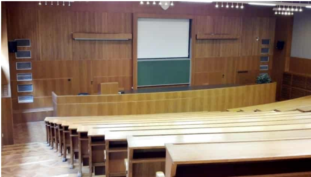
Figure 6: University lecture hall with the vents for supply air
