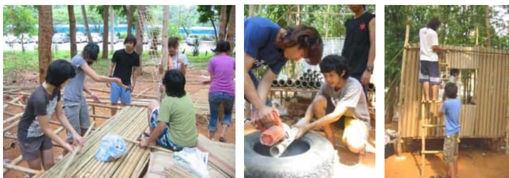
Figure 7. Students learn from their daily construction works
