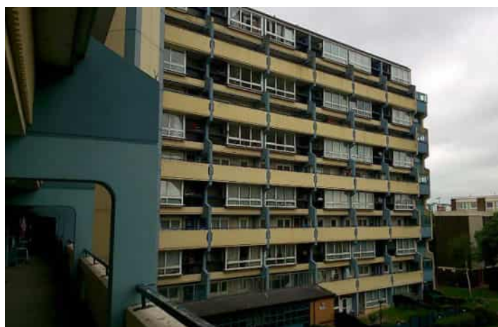
Figure 1. The rear façade of Wilmcote House before refurbishment
