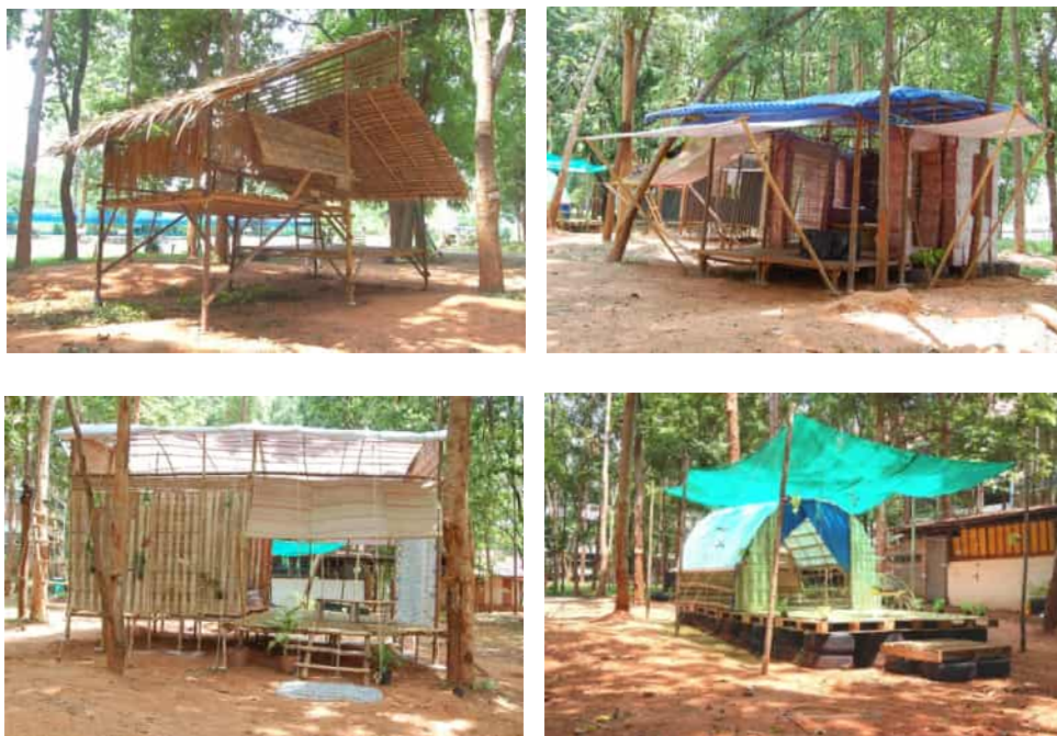
Figure 8. Four final shelters
