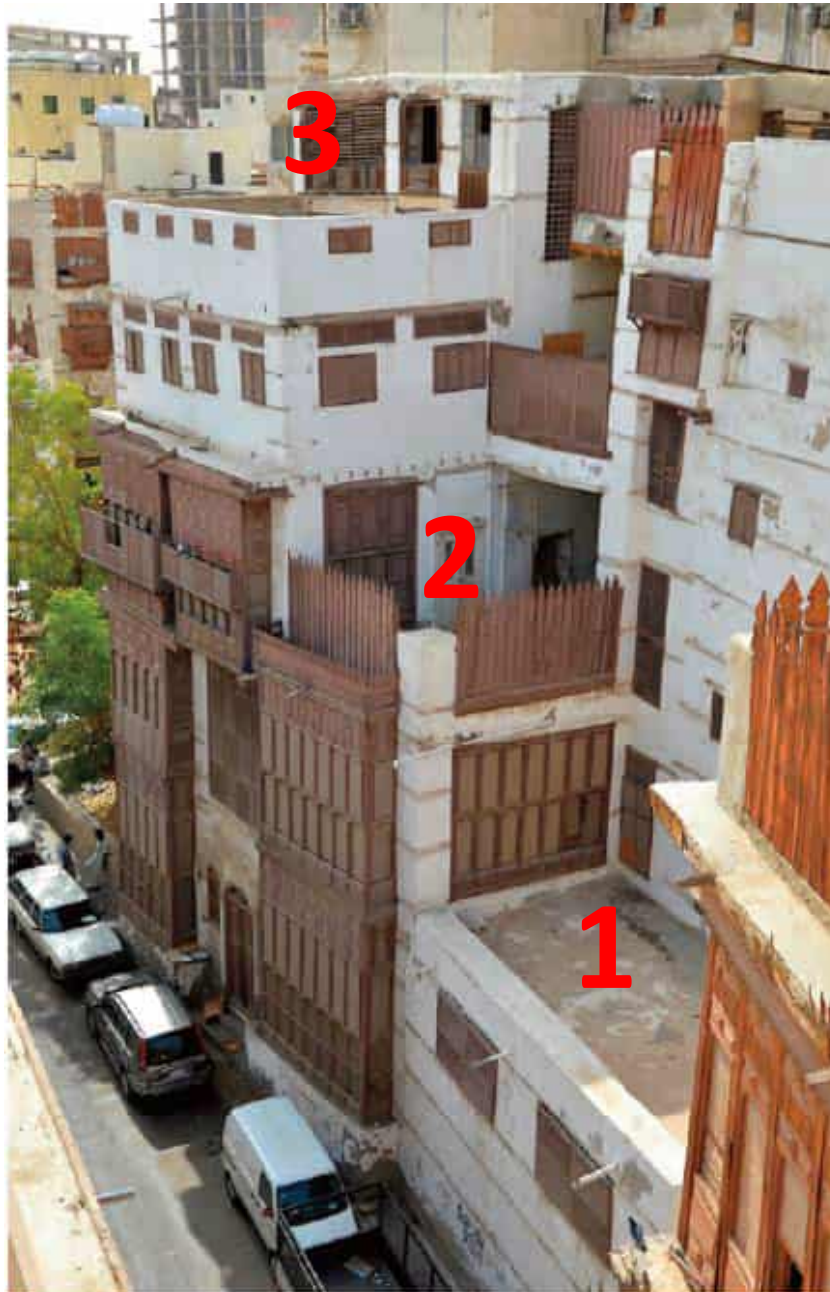
Figure 9: Open spaces appeared in the upper levels of the traditional district with different forms based on the required degree of residents' privacy. For example, number [3] is a private outdoor space for the family, so it was surrounded by walls to ensure privacy for household and neighbours as well. Source: [12]
