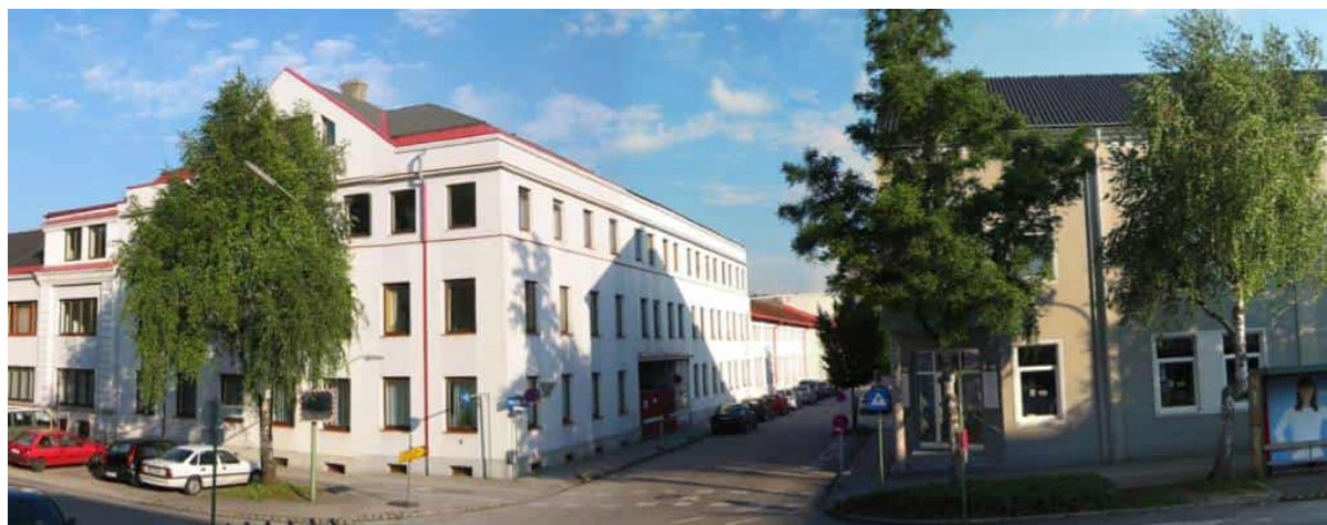
Figure 8. corner Bahnhof/Froniusstrasse before refurbishment
