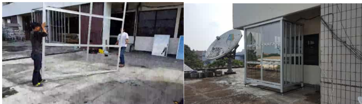
Figure 1. Building panel on double skin façade testing model
