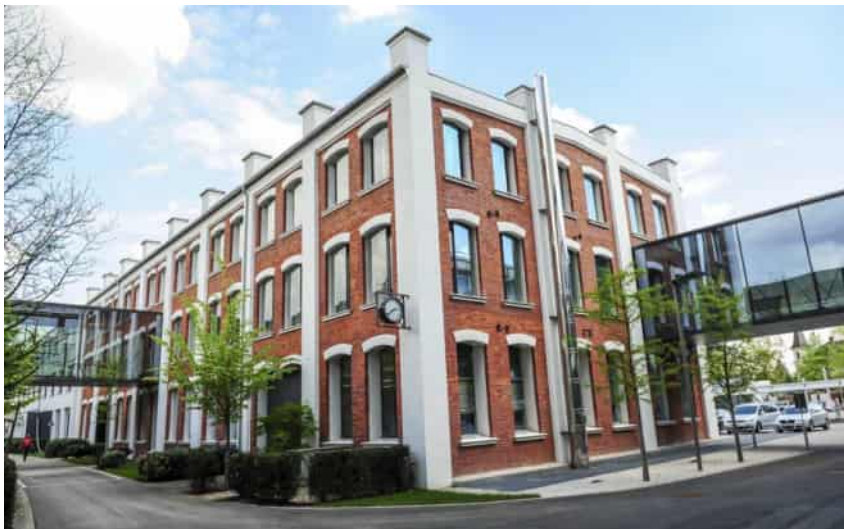
Figure 28. brick stone building connected
