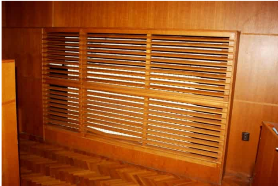
Figure 9: Big university lecture hall with the column radiator
