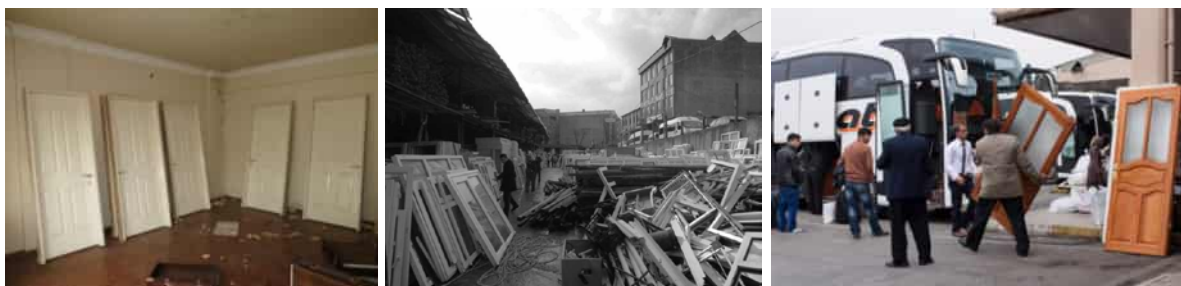
Figure 13. Dismantling of the doors for reuse before destruction in Fikirtepe [14].
