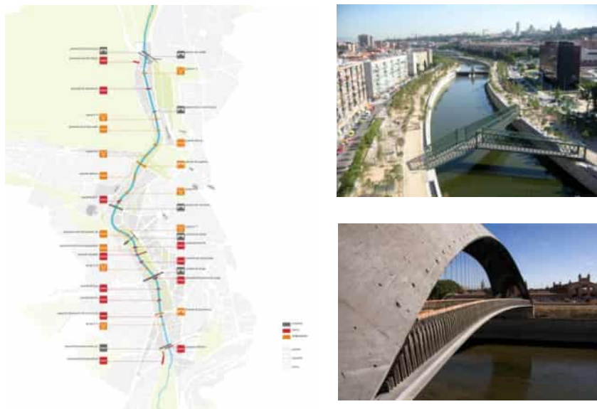
Figure 11. The total 33 bridges
