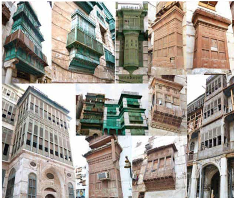
Figure 8: Different styles of Roshan as they appeared on the houses' facades in the traditional district. Source: [8, 12, 17]
