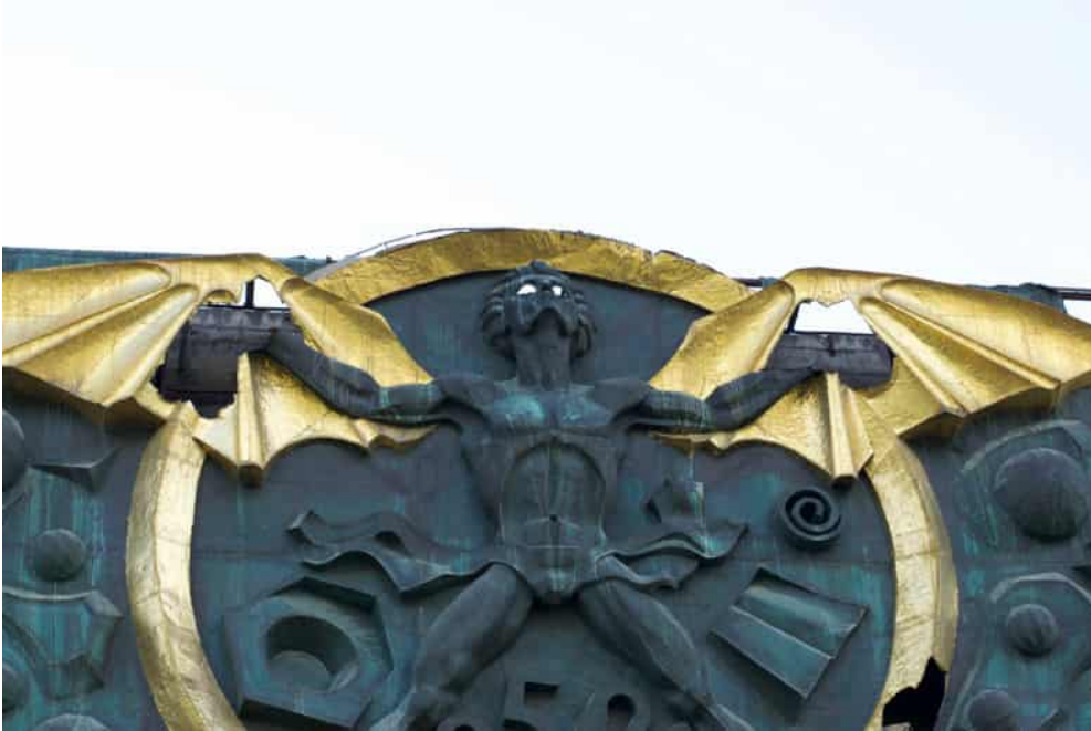
Figure 1: Sculpture on the façade of the former Industrial Pedagogical Technicum in 2017
