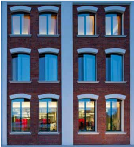
Figure 20. extract brick stone building
