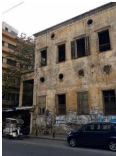
Figure 4. Photo of an abandoned traditional two-storey building in Ras el Nabeh region, Beirut (photo available at Beirut Heritage group, archived in 2017)
