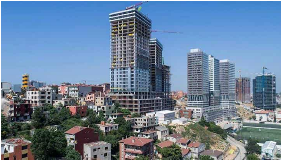
Figure 16. High-Rise Housing Layer of Fikirtepe [URL 4]
