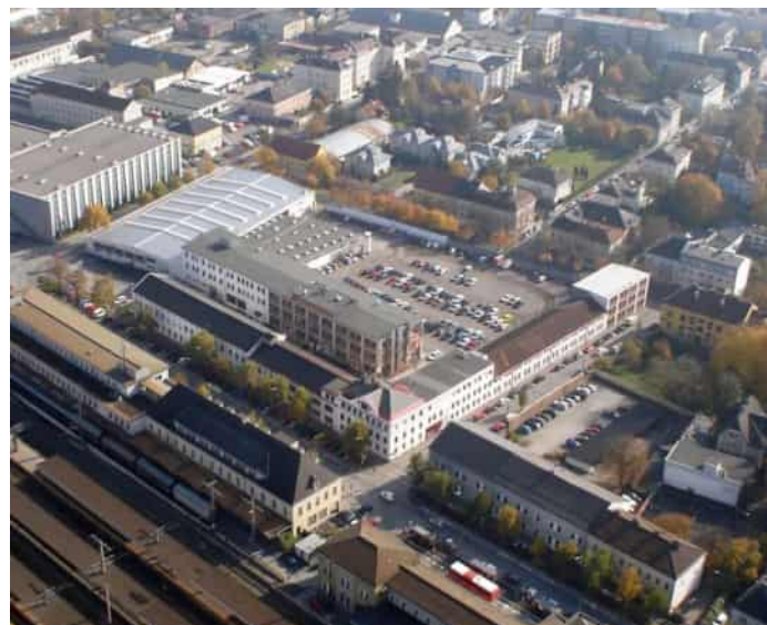
Figure 4. stock before refurbishment
