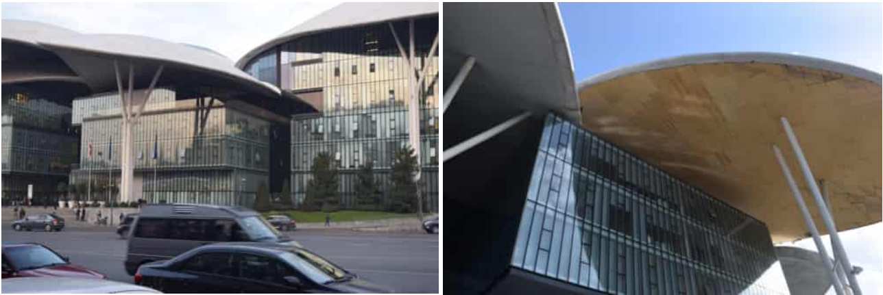
Figures 3 and 4: The Public Service Hall by Fuksas completed in 2012
