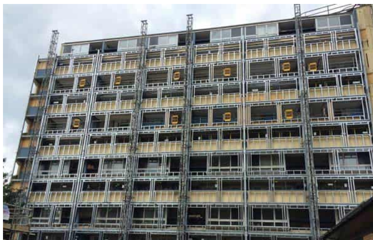
Figure 3. Steel framework and grillage on the rear façade of Wilmcote House
