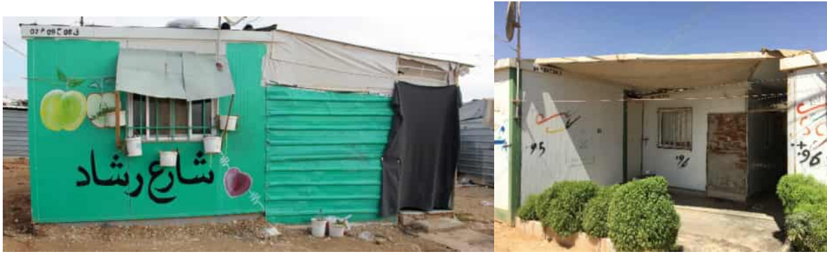
Figure 5: Improved shading solutions and extensions. Notice sharp edges could be dangerous for children
