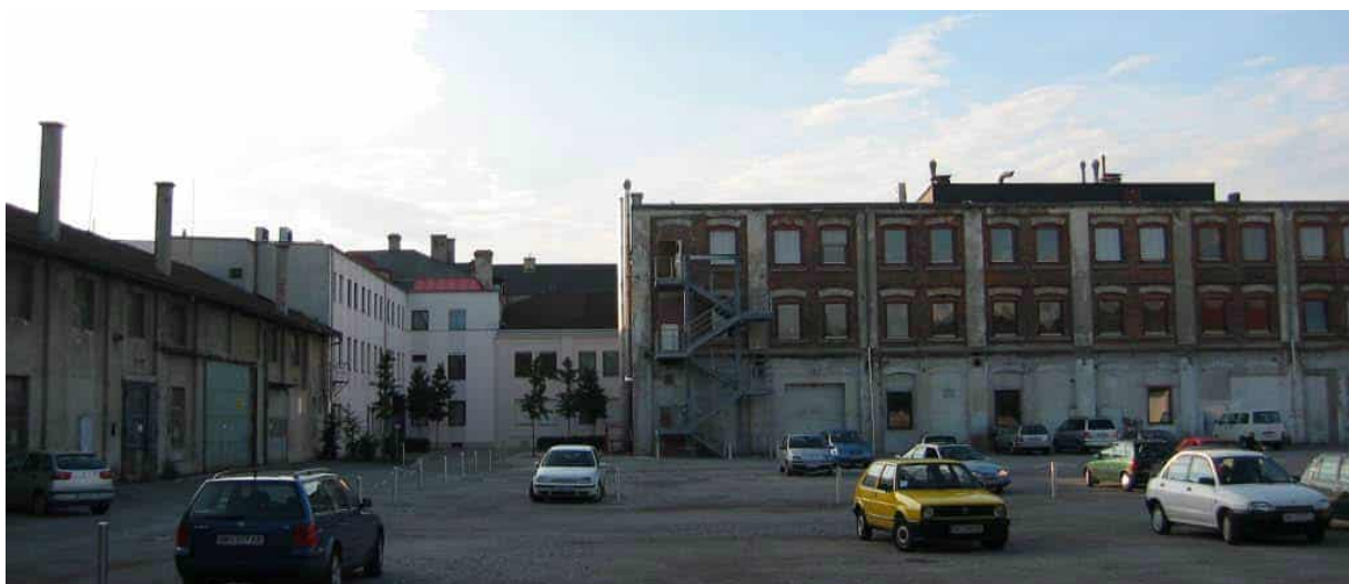
Figure 5. court before refurbishment
