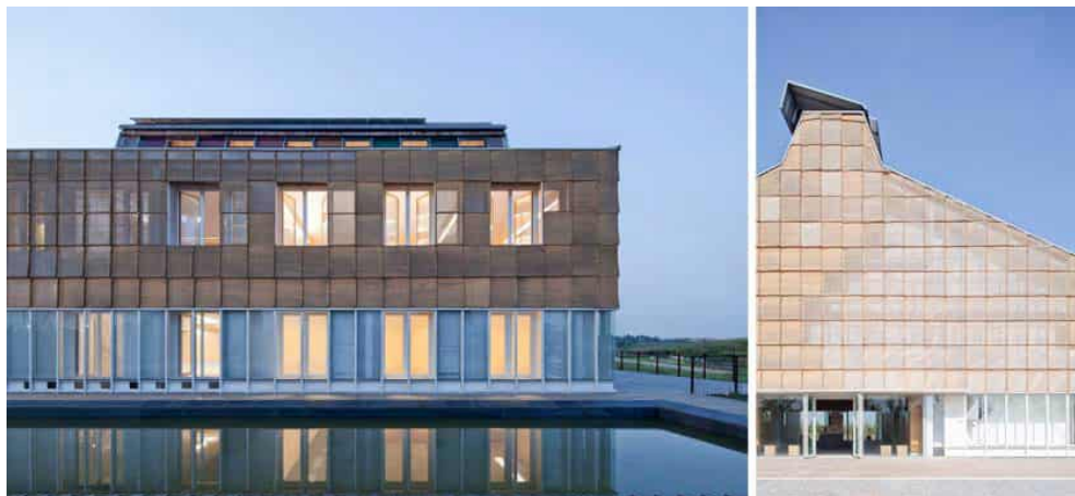
Figure 4. Application of DSF prototype on first floor of THE Studio
