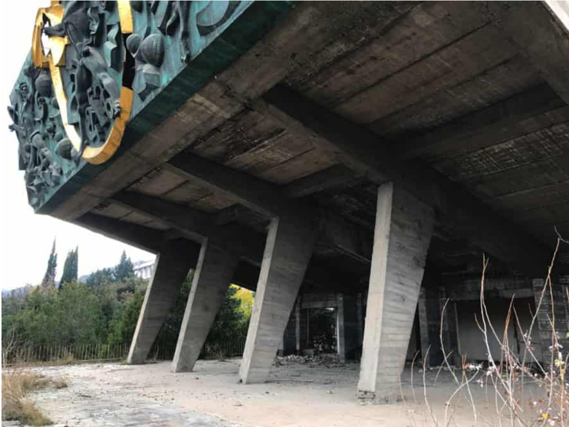
Figure 6: Industrial Pedagogical Technicum Theater Terrace
