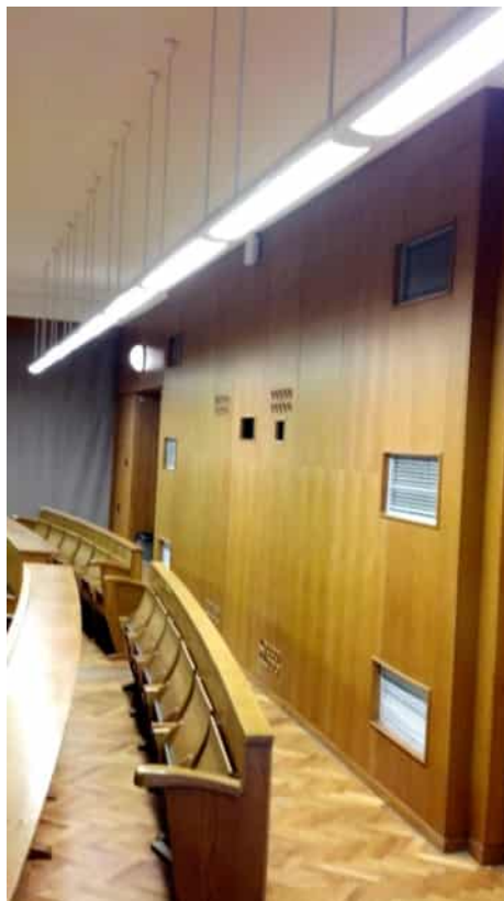
Figure 7: University lecture hall with the vents for extract air
