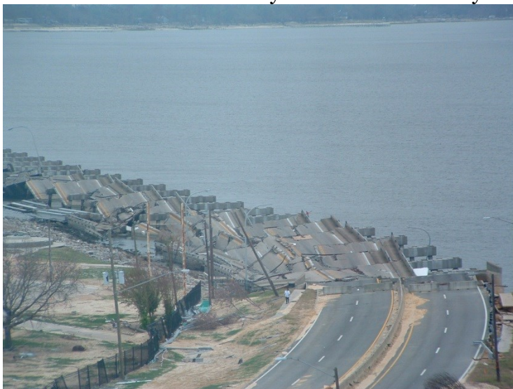
The bridge that linked Biloxi with Ocean Springs pre-Katrina. Mississippi would decide how federal funds would be spent to build its replacement.
