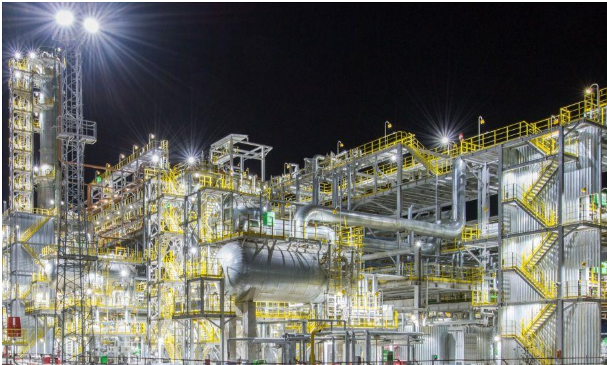
Digital Refinery Project – Central Asia
