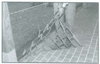
Do not stand or walk on the sections of pavement where the stencil has been removed because the chips of colour will stick to the surface of the pavement and then will be difficult to remove. When the stencil has been removed, use a mechanical blower to remove the remaining chips of colour hardener, and then with a stiff bristle broom, brush clean the entire area. At this time all masking and any "overspray" can be removed.
