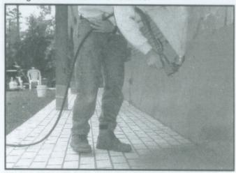
Coverage for each 20kg bag of SPRAYCRETE is normally 10-12 m2 subject to weather conditions and operator skill. Fill spray gun hopper with SPRAYCRETE mix and select correct position to start application, when applying SPRAYCRETE rotate the spray gun in a circular motion, this technique will achieve a good even texture. The texture and consistency of SPRAYCRETE may also vary according to the distance of the spray head to the concrete pavement surface.
