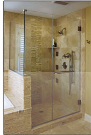
Leaks are minimized.
