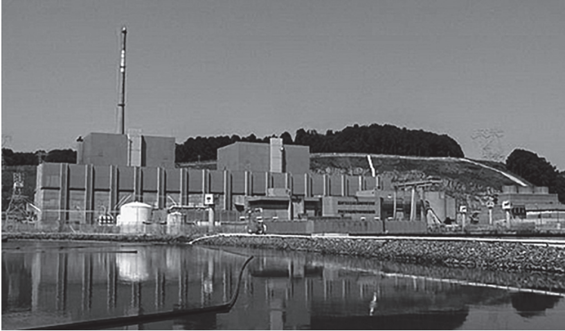
Peach Bottom Atomic Power Station
