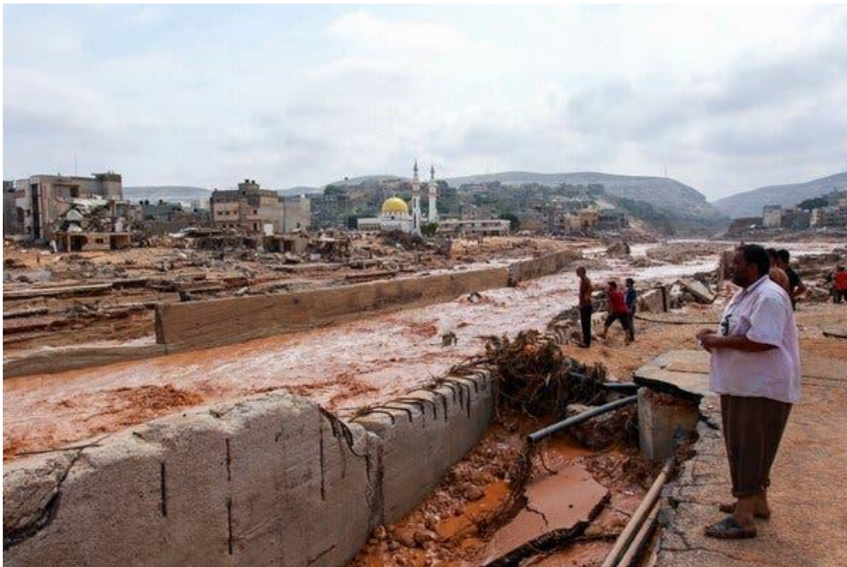
Damage caused by flood in Derna city of Libya on September 11, 2023, Photo Credit: New York Times
