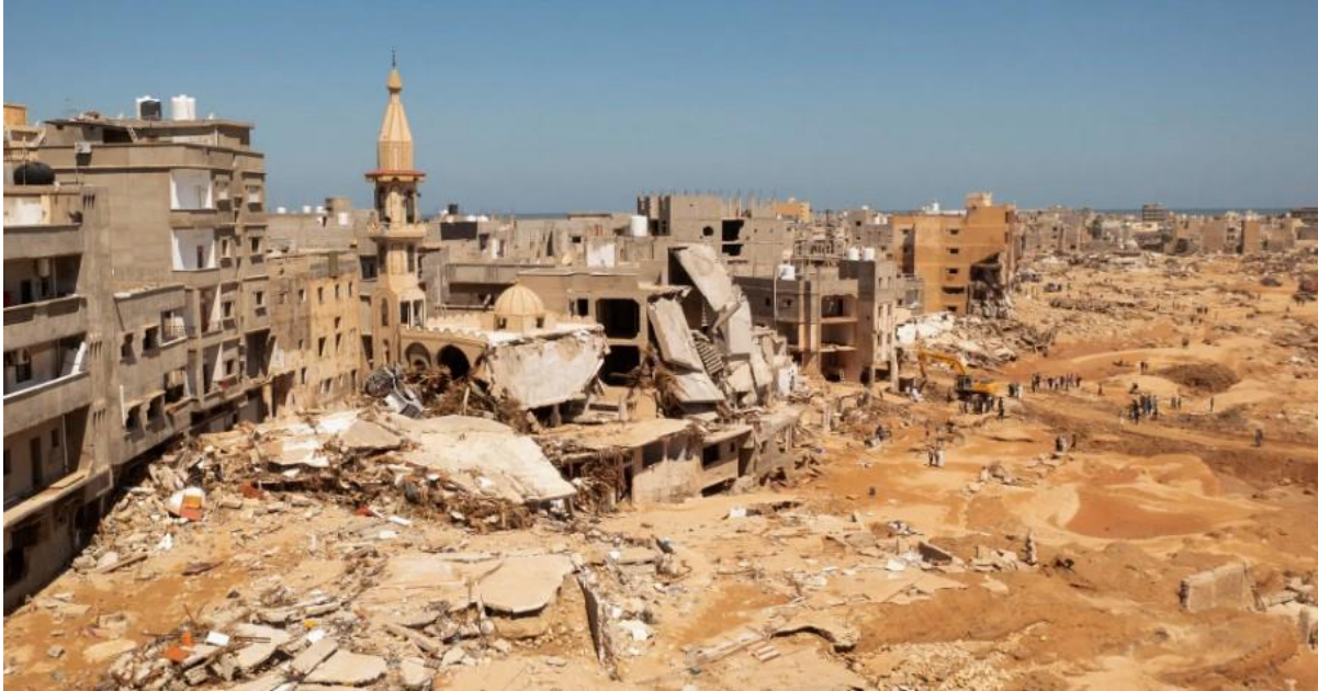
Derna, Libya, after torrential rains burst through two dams near Derna, on Libya's northeastern coast, destroying much of the city. Photo Credit Ayman Al-Sahili/Reuters
