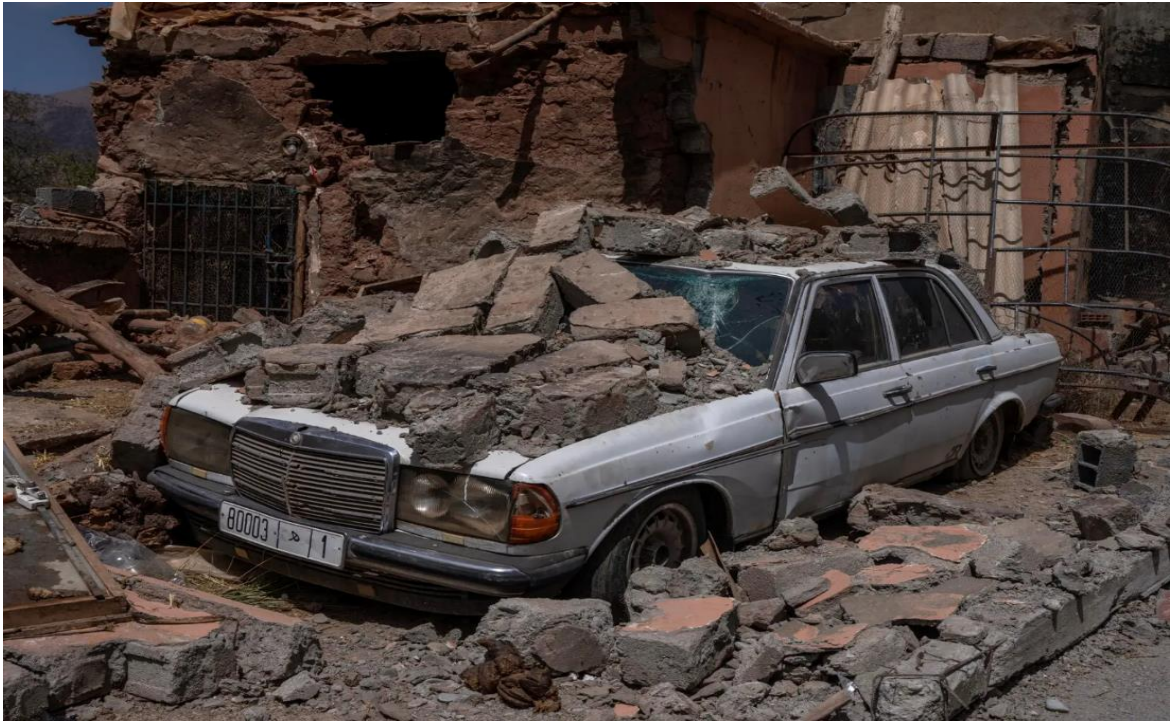
The earthquake brought massive destruction as this car sits buried beneath the rubble left behind. Nariman El-Mofty/ The New York Times
