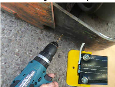
Drilling for End Caps
