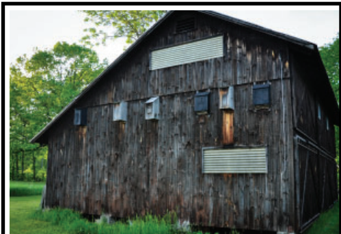
Bat houses are a great alternative for bats you need to evict from your home, but they do require some maintenance in the late fall or winter to clean out abandoned wasp nests and repair any leaks.
