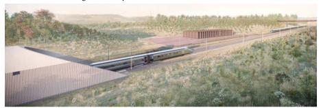
Following our comments raised at the Key Design Exhibits last March the hardstanding for the compound will now be comprised of a light grey/buff coarse stone surfacing to blend into the surrounding railway cutting and Chilterns AONB.
