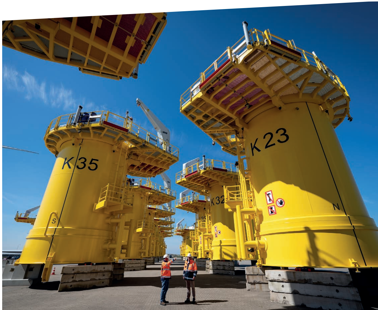
The handling of various components for the offshore wind park Kaskasi is carried out at the Buss Terminal Eemshaven in the Netherlands
